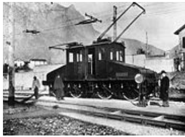
The world's first AC locomotive in Valtellina (1898-1902). Power supply: 3-phase 15 Hz AC, 3000V, (AC motor 70km/h). It was designed by Kálmán
