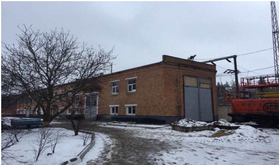
Figure 1. Traction substation No. 18, Zmiiv.
